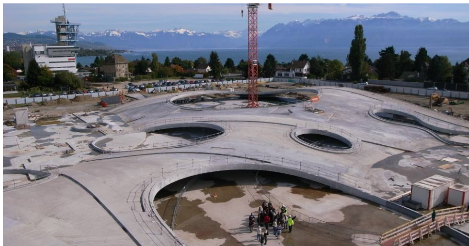
Figure 2: view on the big shell after removing of the formwork
