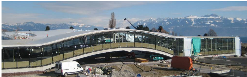
Figure 1: view to the eastern façade during construction
