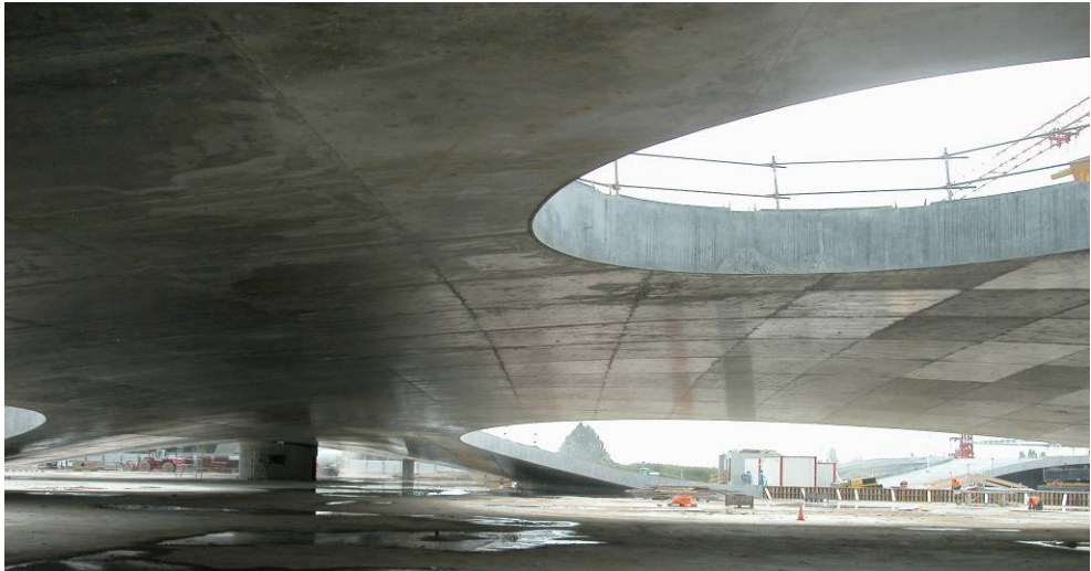
Figure 17: big shell after removing of the formwork
