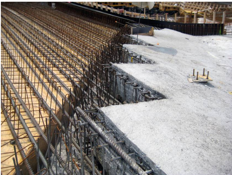
Figure 16: construction joint at the shell bearing
