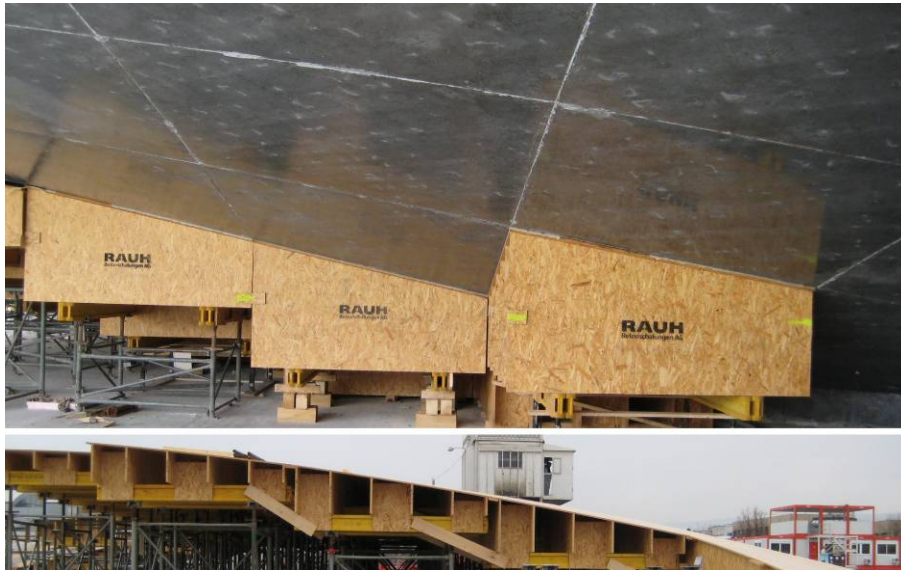
Figure 7: formwork tables on sight; after and before concreting
