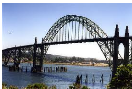
Yaquina Bay Bridge (McCullough, 1936)
