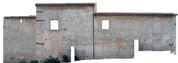
Fig. 7. Photogrammetry of the lateral façade (Source: the authors).
