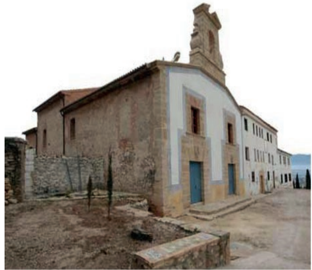
Fig. 6. Photograph of the convent from the north corner (Source: the authors).
