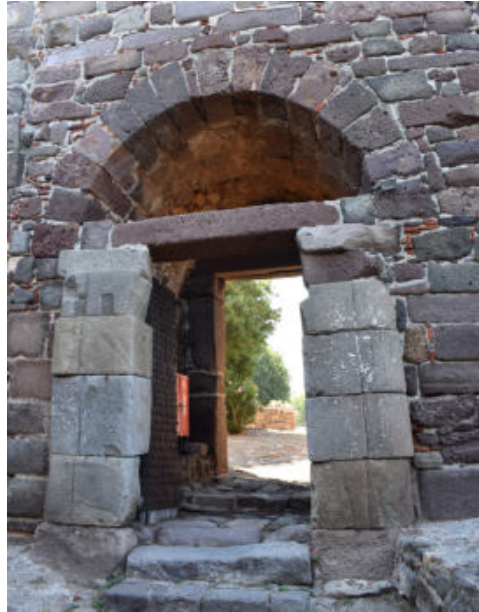
Fig. 6- The entrance gate after its modification possibly in the 15 th century (photo by Klimis Aslanidis, 2020)
