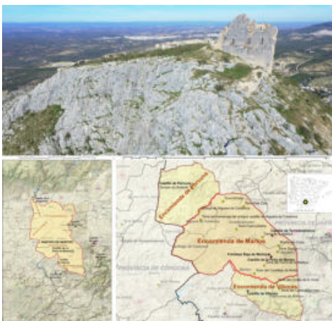
Fig. 1- (Top) Aerial view of the Castle of La Peña from SW. (Bottom right) Territorial organization of the Commands of Martos, Viboras and Porcuna during the Late Middle Ages and their main defensive structures. (Bottom left) Territorial border on the 1785 geographical map of the district of Martos (photos and graphic elaborations by the authors)
