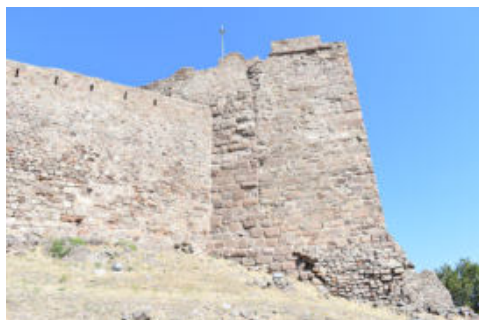
Fig. 9- The northeast tower 7, added to a previous smaller tower. (photo by Klimis Aslanidis, 2020)
