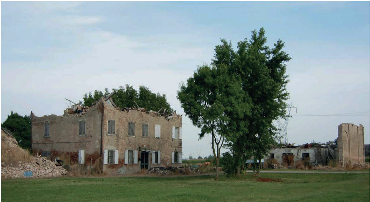
Figure 1 | San Giacomo Roncole in the district of Mirandola, Modena. In the historic courtyard, the stable-barn and the dwelling collapsed due to wall-roof interaction.
