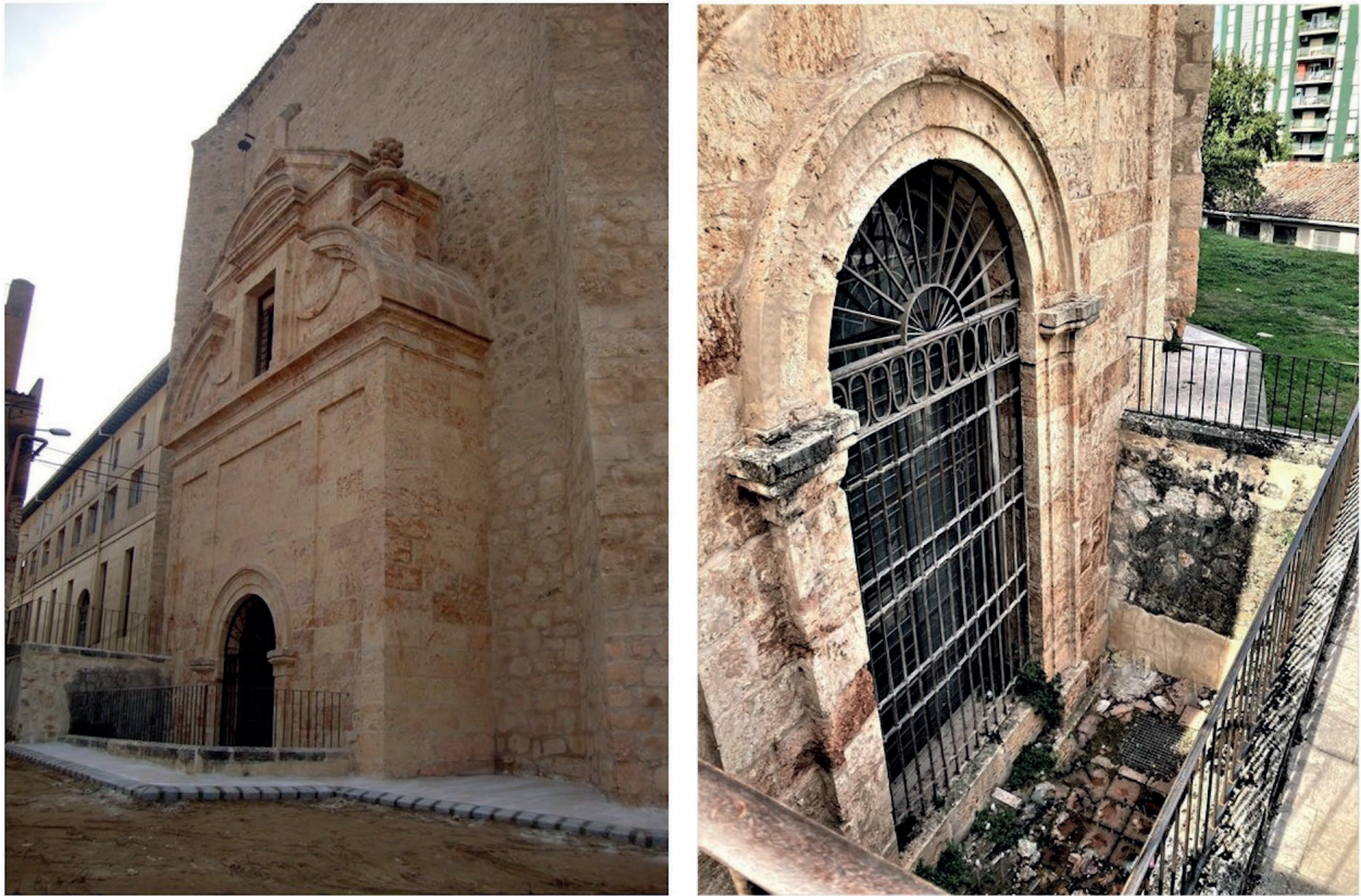
Fig.13. Rear façade of the Pantheon. Photographs: The author.
