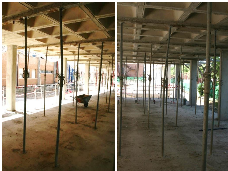
Fig. 1. Shore buckling during the construction of a building structure.
